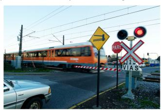
The E-300 level crossing is "fail-safe" SIL-4 according to CENELEC standards, allowing different configurations both wired or radio communications.
